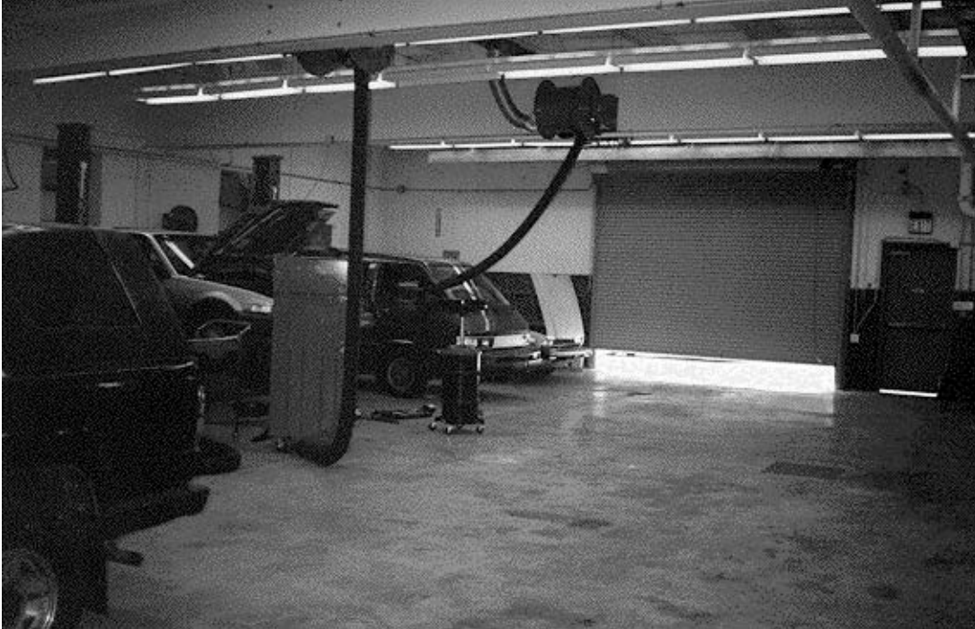
Interior view of existing AutoTech Center
