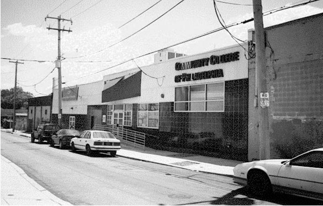
West Philadelphia Regional Center, Ludlow Street facade, looking southeast
