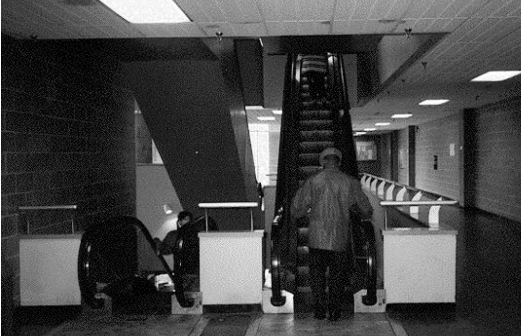
Existing escalators in Bonnell Building frequently break-down, are noisy, and block views through the space
